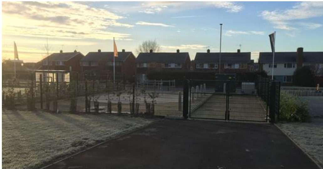
Figure 3: Typical pumping stations appearance
